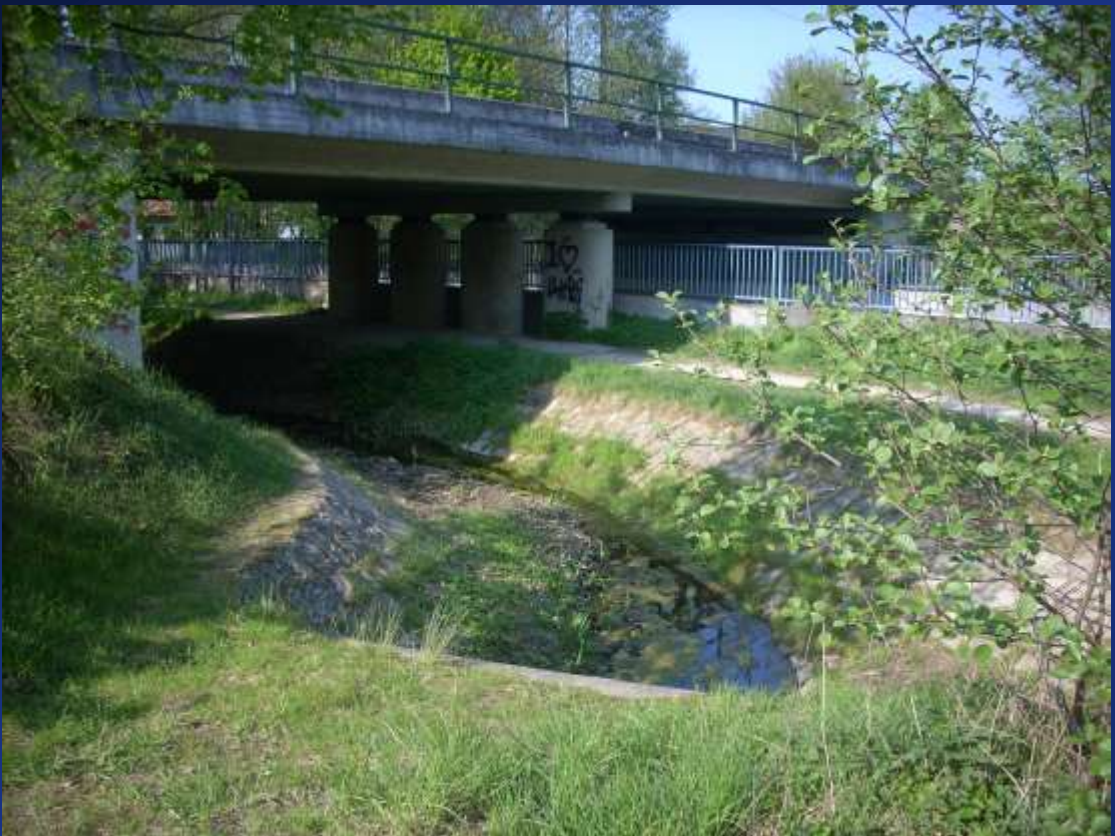
Steinbach, Stat. km 5+800
