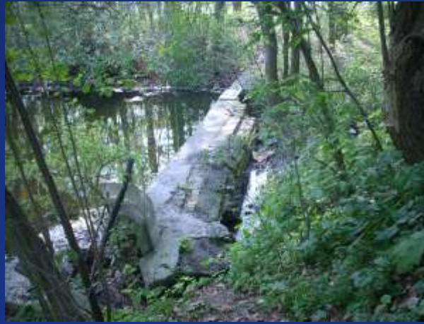
Steinbach, Stat. km 8+400
