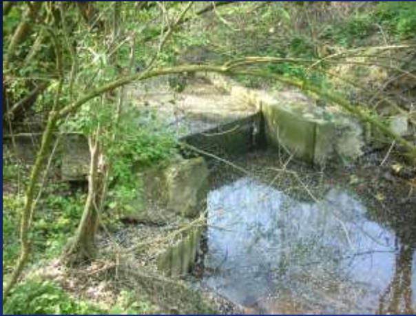
Steinbach, Stat. km 6+050
